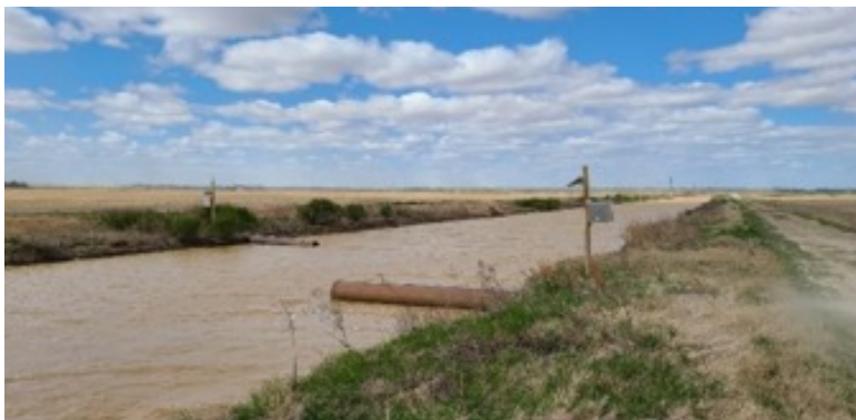
Figure 1c tailwater recovery ditch after heavy November rains. (Almost all the runoff pipes were under water at this point, often backing up into the field, making it difficult to record flow rates).
